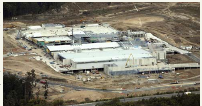
Massive Orion Shopping Centre under construction is now open
